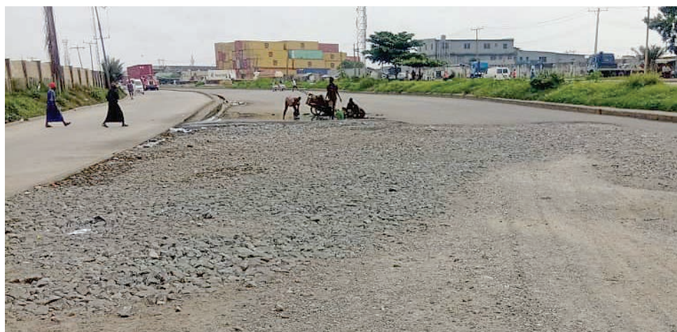
National Theatre Bridge section of the road
