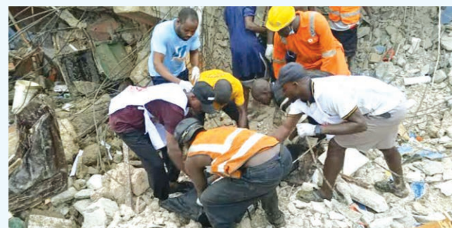
Rescuers during Alakija building collapse in Lagos
