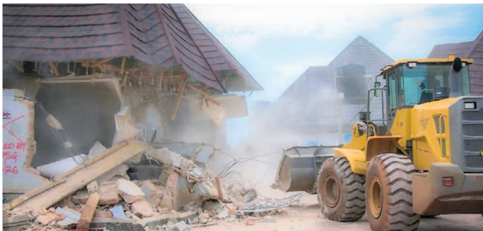
Edo officials during the demolition... yesterday
